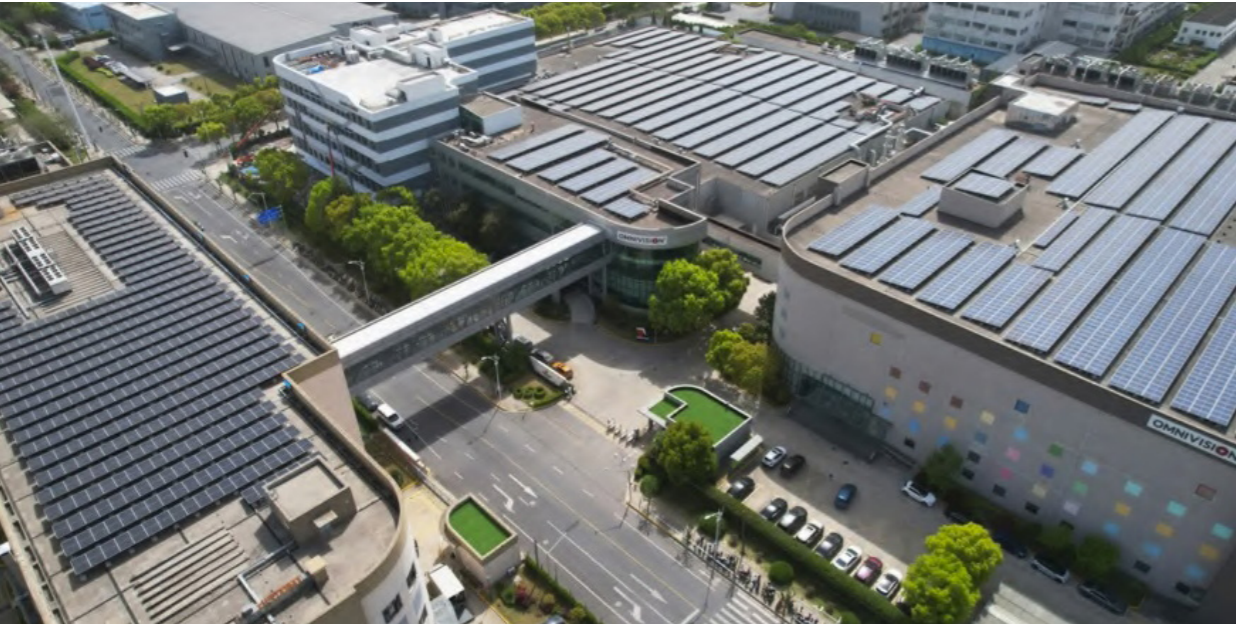
▶ Rooftop photovoltaic power generation system at the Shanghai Songjiang Park
